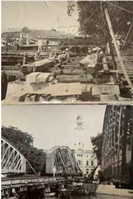
Photographs of Anderson Bridge under construction (1908 – 1910)
